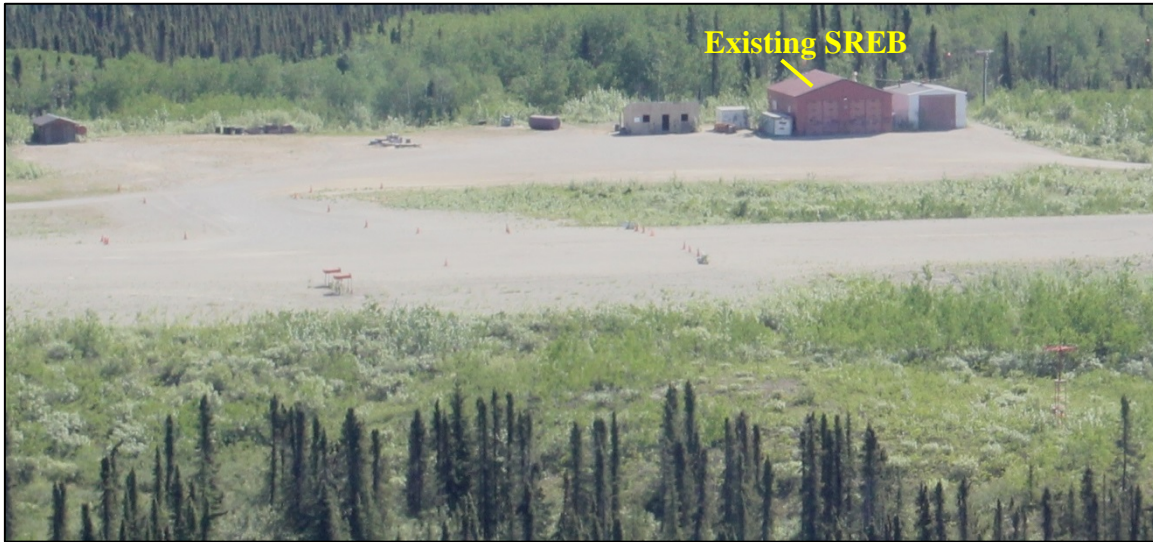
FIGURE 2: AMBLER AIRPORT APRON (DOT&PF)
