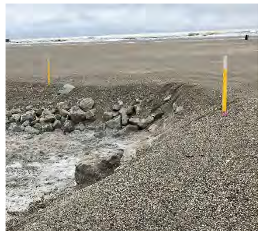
Exhibit 1 – Drainage ditch and culvert within the secured area.
